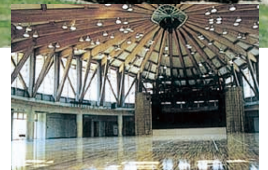
Exterior and Interior of Wooden Dome Made with Large Sectional Laminated Timber
