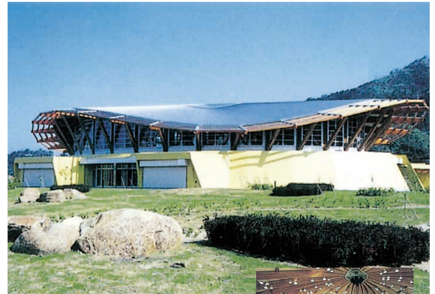
Exterior and Interior of Wooden Dome Made with Large Sectional Laminated Timber
